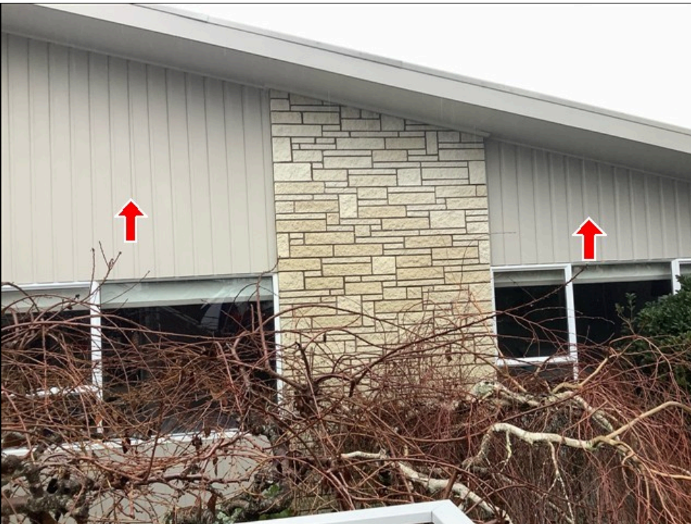
3.2 Item 3(Picture) Asbestos Sheets In Some Areas Around The House
