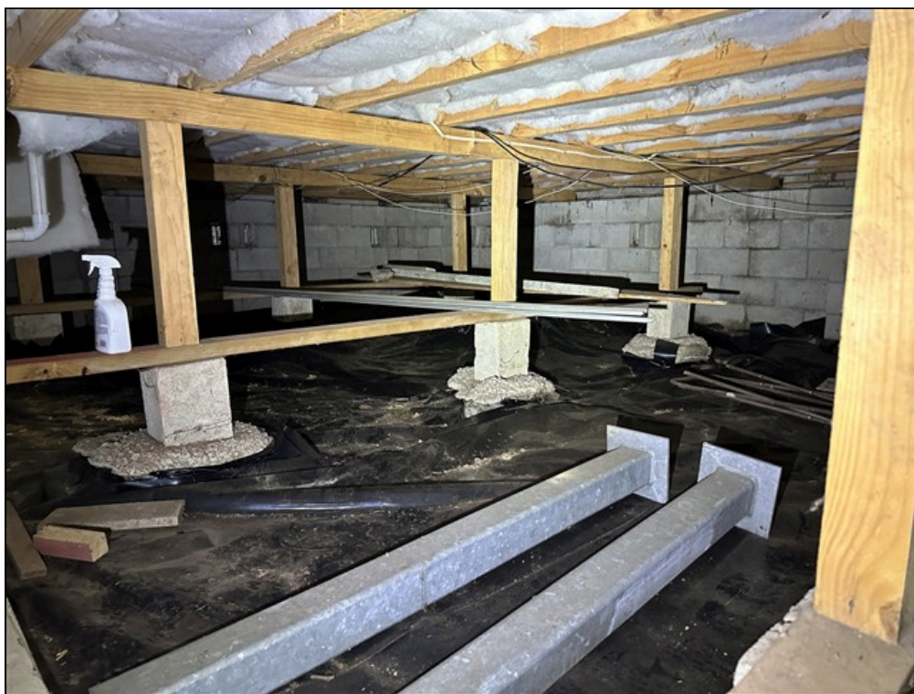
4.3 Item 1(Picture) Some Soil Has Dropped From Around Certain Piles
