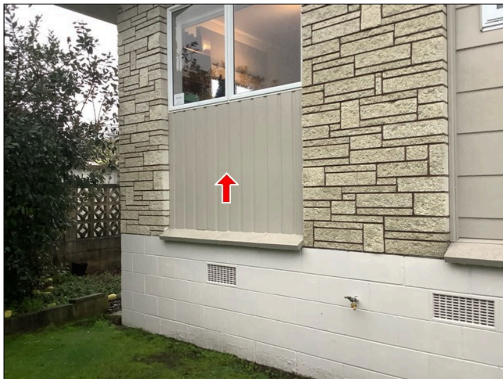
3.2 Item 4(Picture) Asbestos Sheets In Some Areas Around The House
