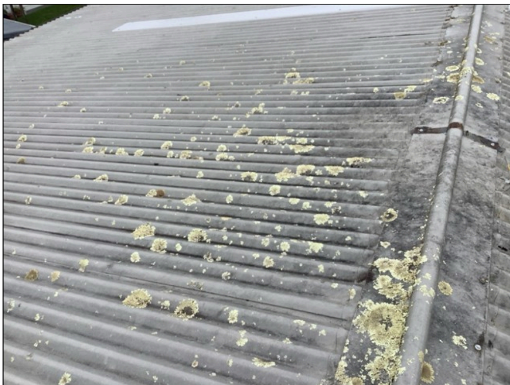
2.2 Item 3(Picture) Lichen Present On The Roof Has Been Treated
