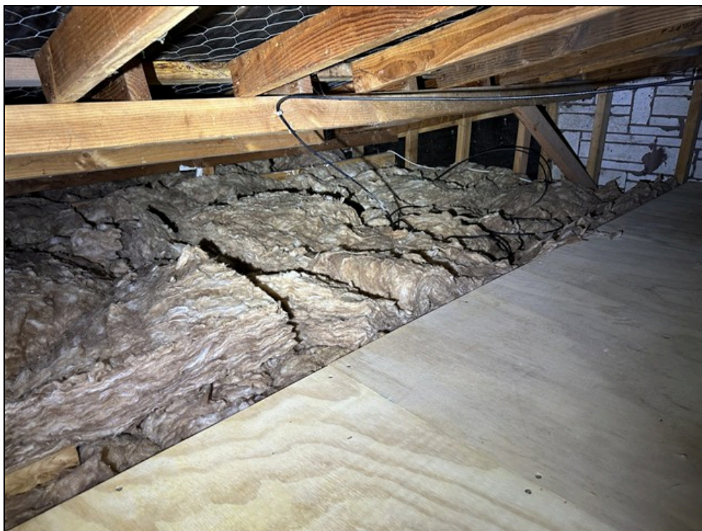
7.3 Item 1(Picture) Earthwool Insulation Installed In The Roof Cavity Area Of The House
