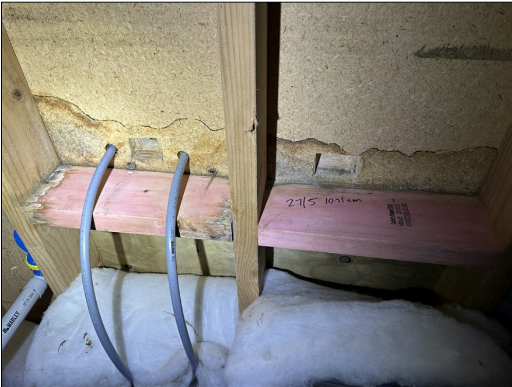
5.19.F Item 8(Picture) Extent Of The Water Leak Underneath The House In The Subfloor
