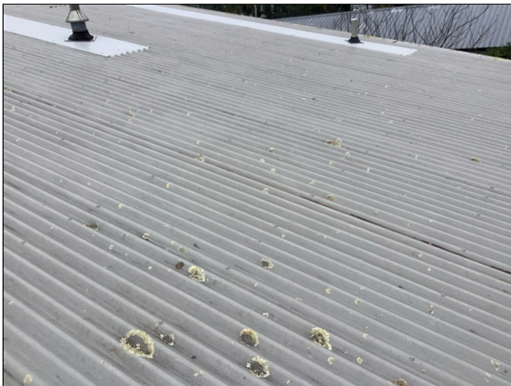
2.2 Item 2(Picture) Lichen Present On The Roof Has Been Treated
