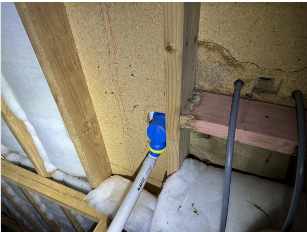
5.19.F Item 9(Picture) Area Has Been Left Open To Ensure It Completely Dries Out
