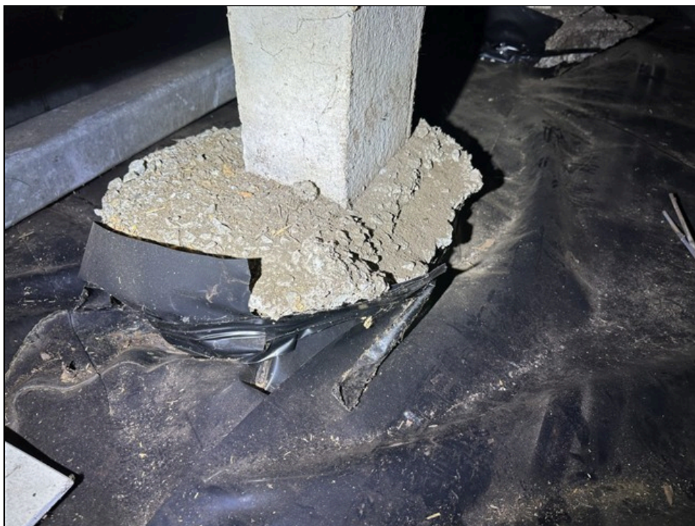
4.3 Item 2(Picture) Some Soil Has Dropped From Around Certain Piles
