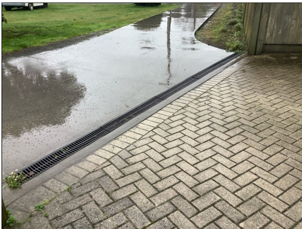
1.8 Item 1(Picture) Channel Grate Drain On The South Eastern Corner Of The Cobble Driveway
