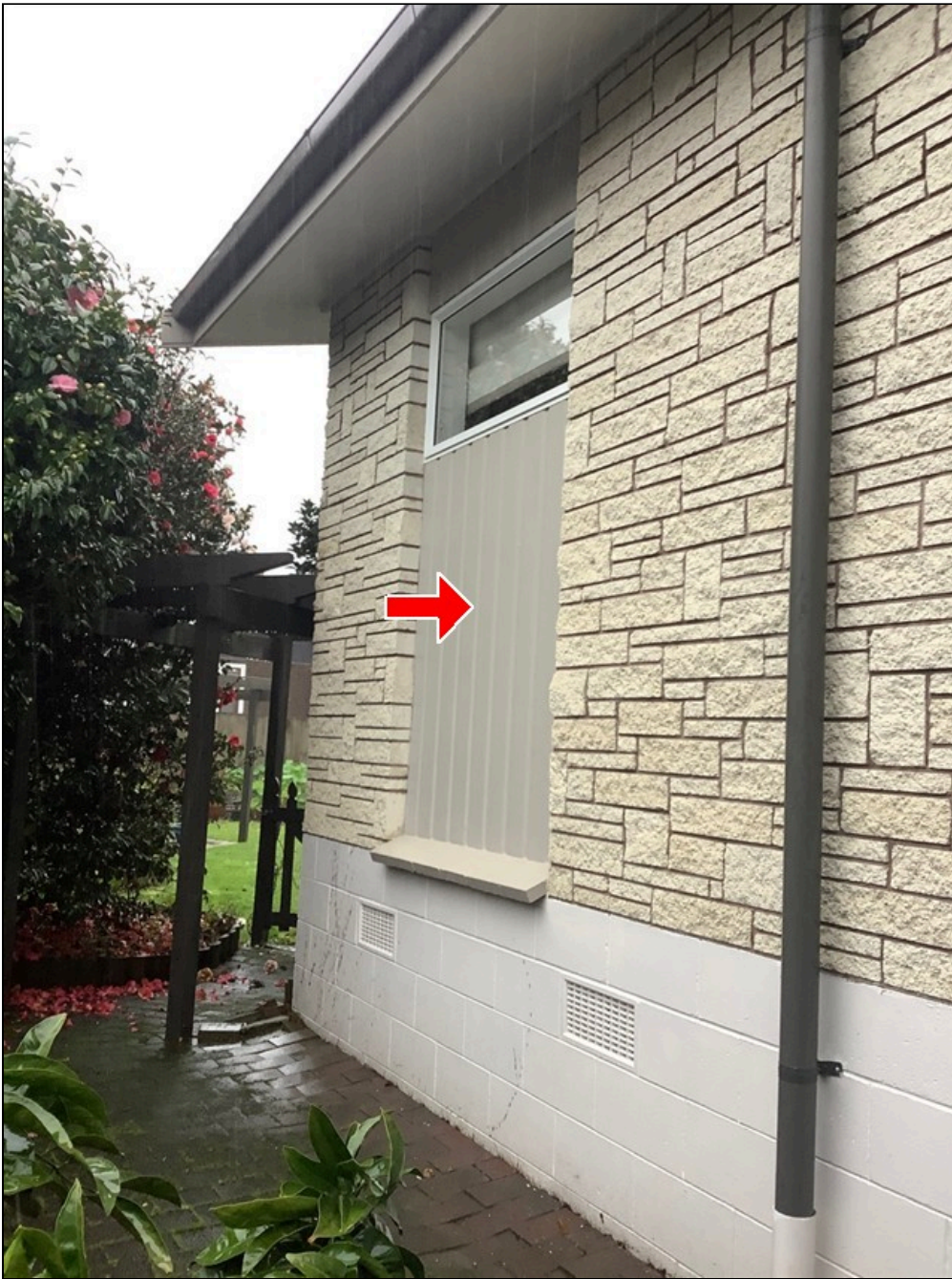
3.2 Item 6(Picture) Asbestos Sheets In Some Areas Around The House
