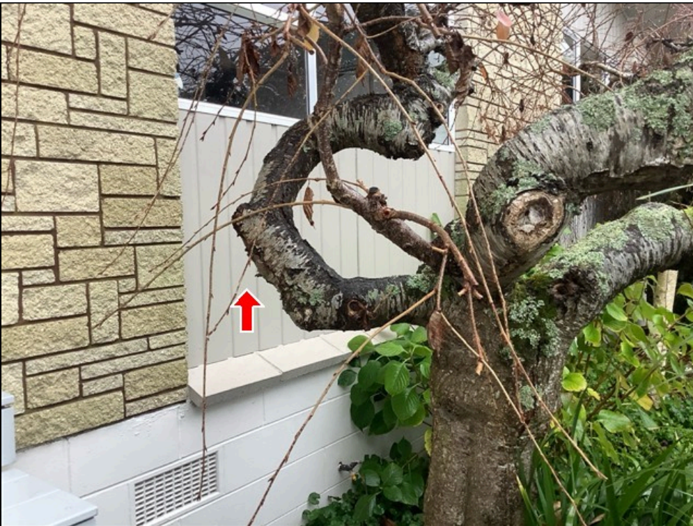
3.2 Item 2(Picture) Asbestos Sheets In Some Areas Around The House
