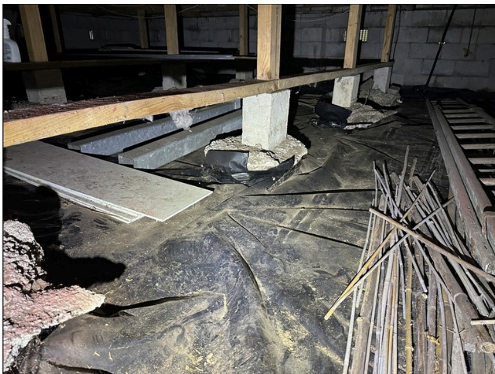
4.6 Item 1(Picture) Ground Vapour Barrier Installed
