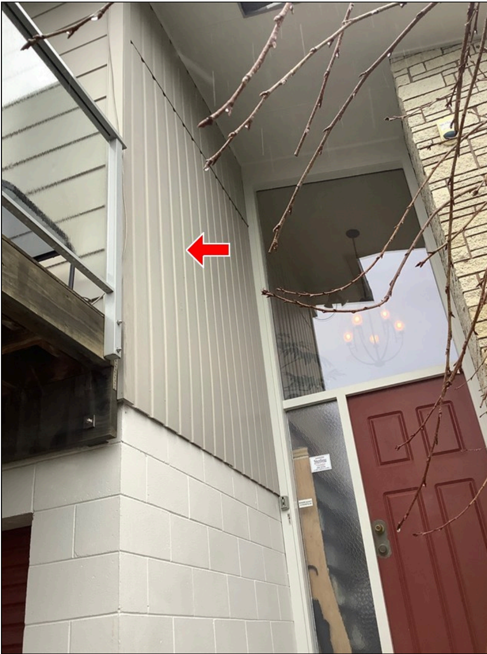
3.2 Item 1(Picture) Asbestos Sheets In Some Areas Around The House
