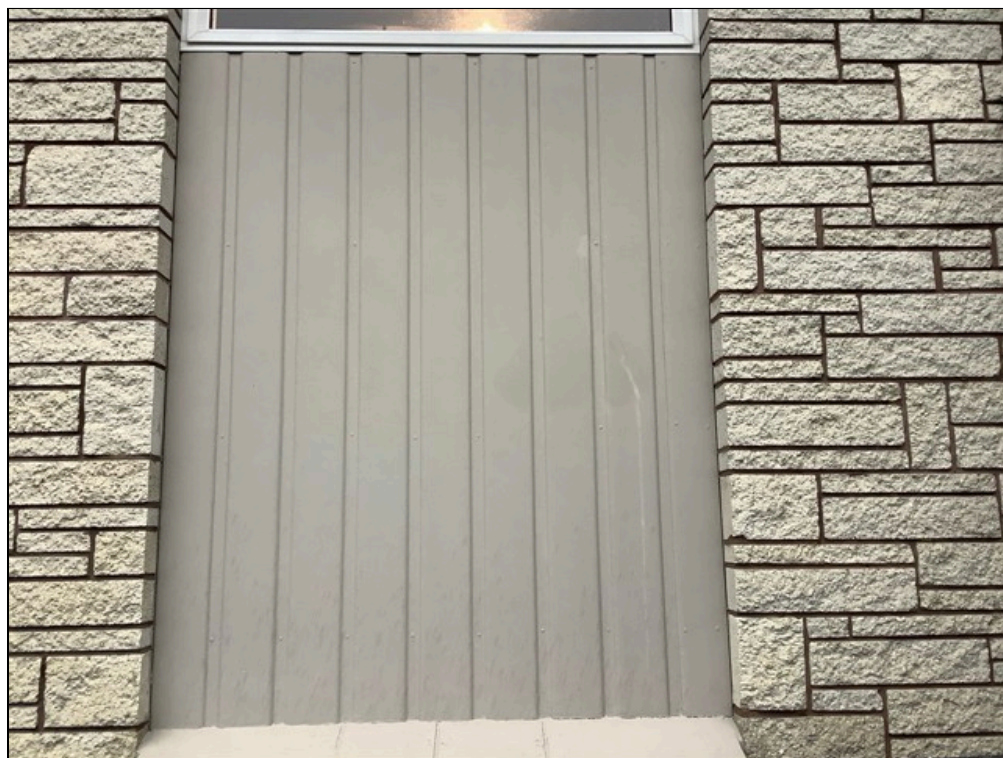
3.2 Item 5(Picture) Asbestos Sheets In Some Areas Around The House
