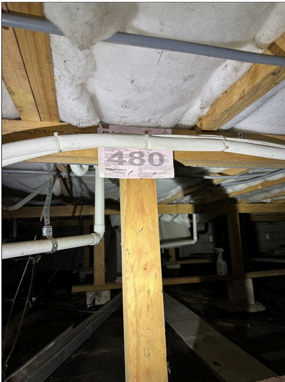
4.14 Item 1(Picture) Polyester Insulation Installed In The Subfloor Area Of The House
