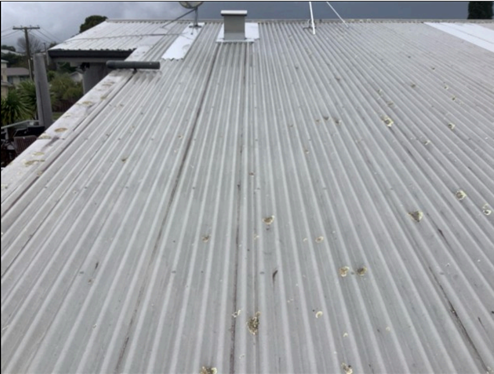
2.2 Item 1(Picture) Lichen Present On The Roof Has Been Treated
